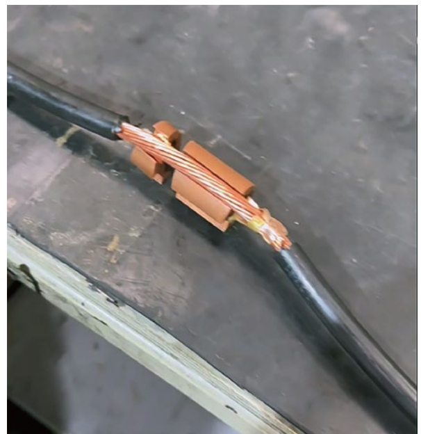
Anode Connector Installation Illustration
